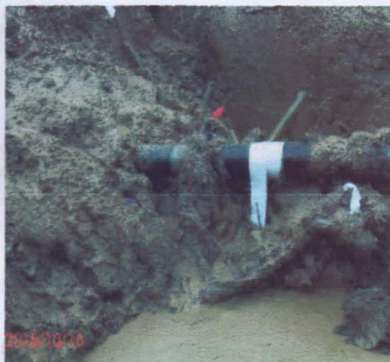
Fig B: picture taken after excavation.
